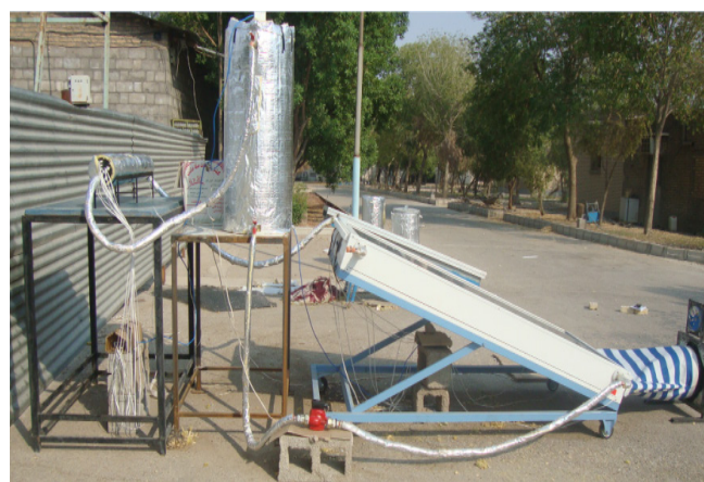
Fig. 1. A view of the solar water heater system
